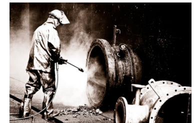
Wikimedia, High-Pressure-Cleaning-of-Heat-Exchanger-Parts, www.wikimedia.org , 2013
